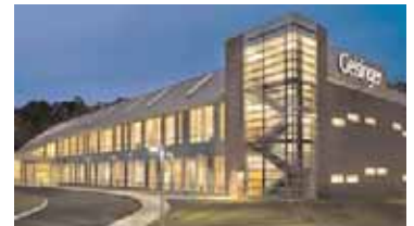
Geisinger Health System earned LEED Gold Certification for its "green" clinic in State College, PA.
